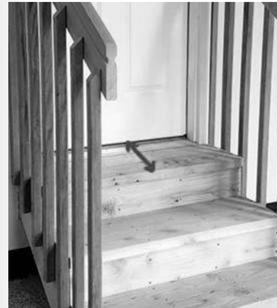
Extended first step landing
